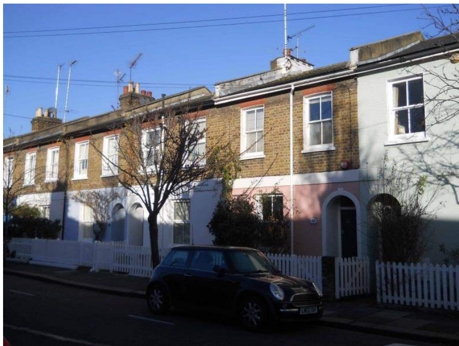
Houses retain their pitched roofs on Redan Street. Picket fences and shrubs in front gardens enhance the appearance and experience at ground level.
