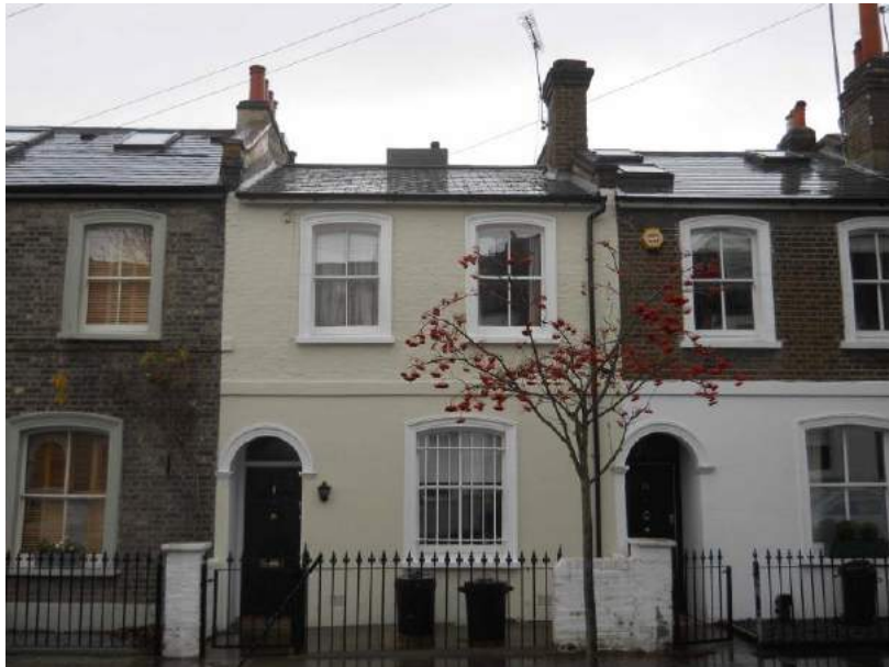
The raised ridge on the roofs to the left and right of the picture accommodates a loft extension. Faroe Road.
