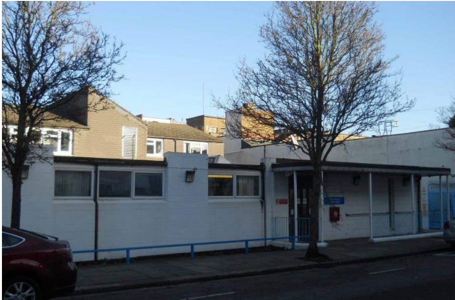
Health Centre Milson Road, an opportunity site.
