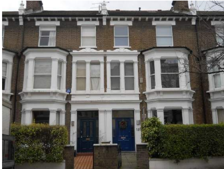
Paired windows above the entrances with stucco scrolled pediments. Nos. 145-161 Blythe Road.
