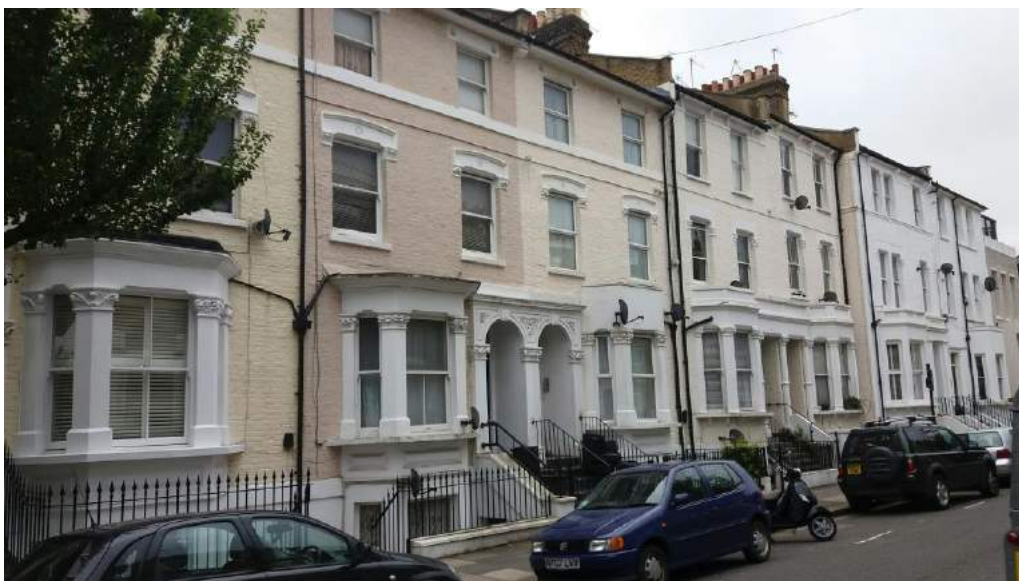
Nos. 107-121 Milson Road.
