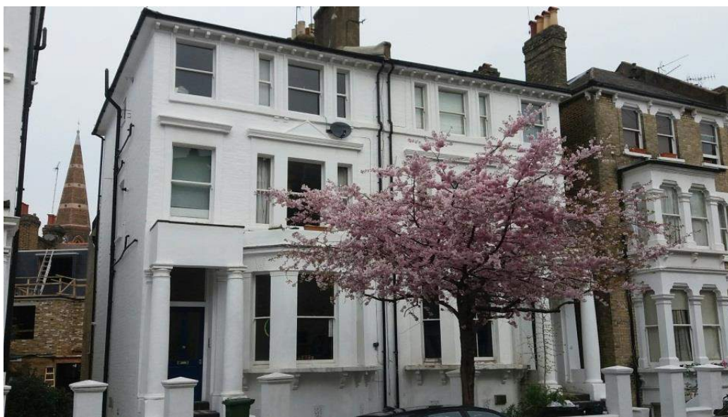
Gault brick no. 61 Netherwood Road on the right and nos. 63-65 centre ground. A glimpsed view of St. Simon's Church spire on the left.
