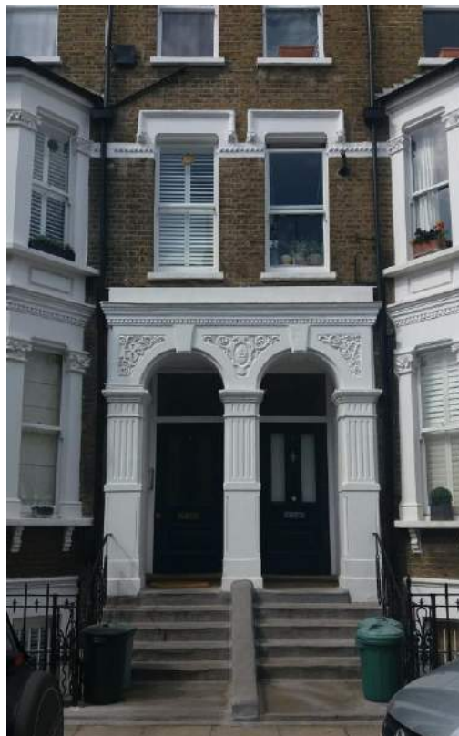
Nos. 2-24 Bolingbroke Road. Richly detailed stucco porches.
