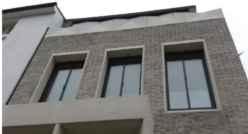
No. 121 Milson Road. Attractive details include deep window reveals, faceted parapet and upper storey glazing.
