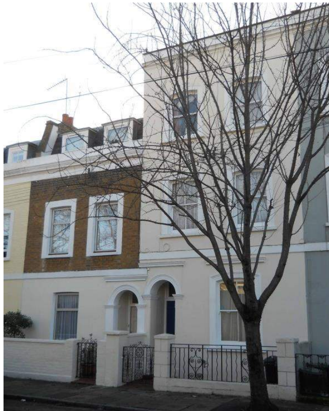
Nos. 28 (right) and 30 Milson Road.
