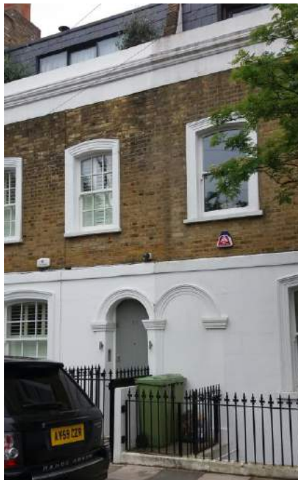
Infilled porch, no. 53 Faroe Road.
