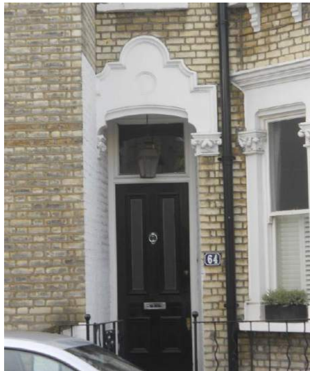
Elaborate stucco pediments, nos. 60-66 Milson Road.
