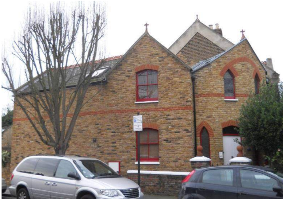
No. 1 Fielding Road turning onto Masbro Road. Attractive red brick soldier courses in window arches and string courses.
