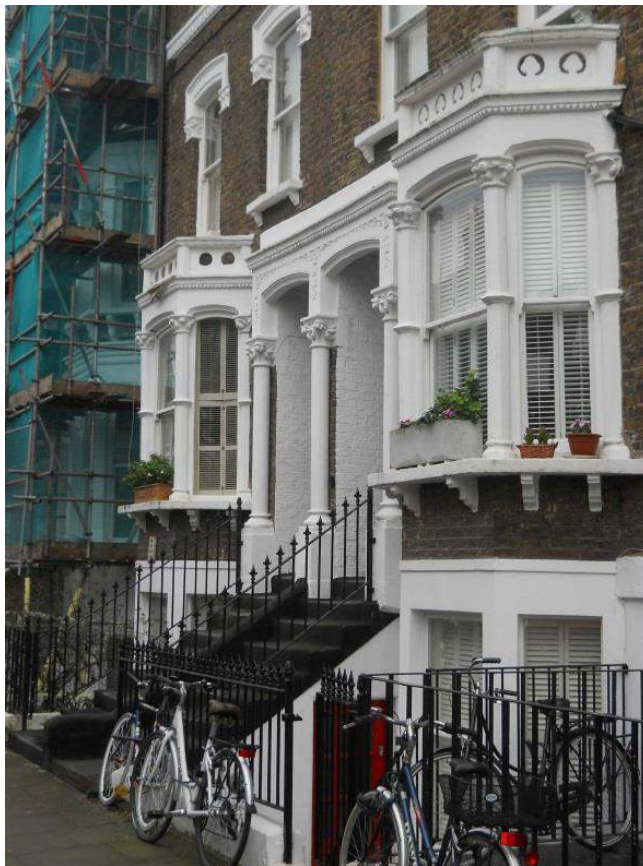
Typical stucco decoration Gratton Road and original railings.
