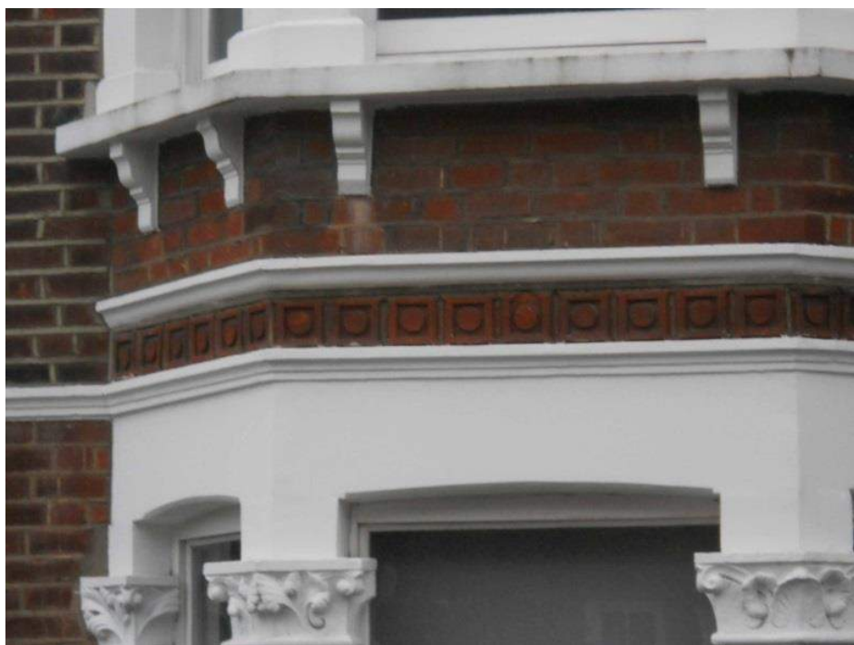
Distinctive moulded brick pattern on nos. 69-83 Bolingbroke Road.
