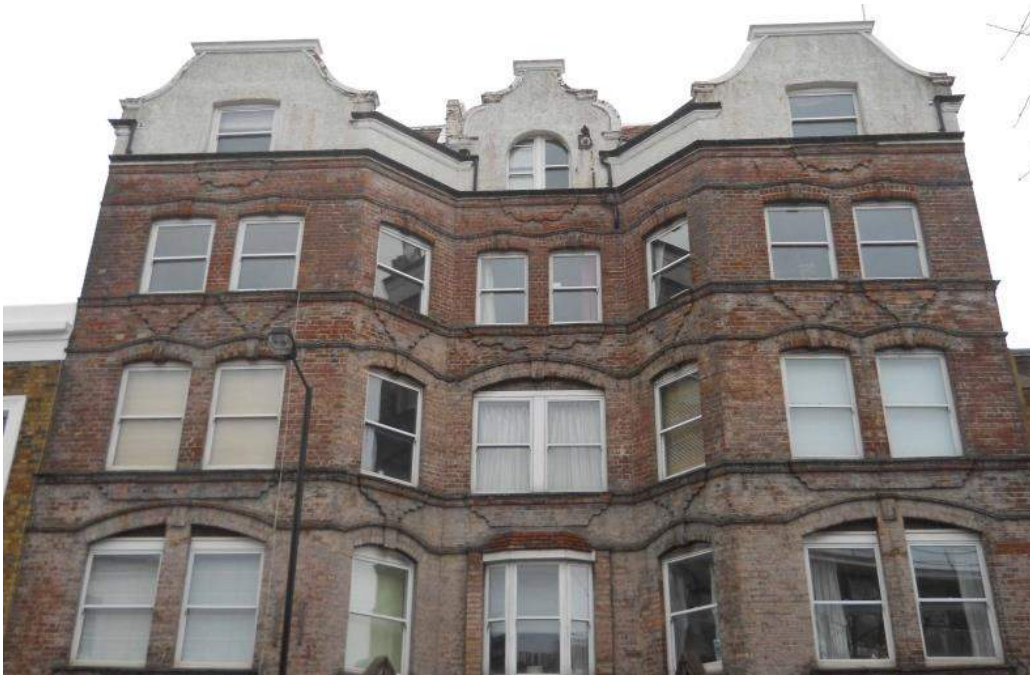
Elaborate brick detailing, no. 112 Blythe Road.
