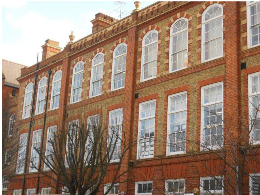
Elaborate cornice and parapet on Addison Gardens Primary School. Street trees along the perimeter enhance its setting.
