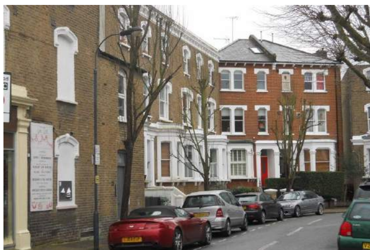
Sterndale Road showing two styles of housing, those with a parapet and those with a pitched roof. One of the large trees that typify the street is visible on the left.
