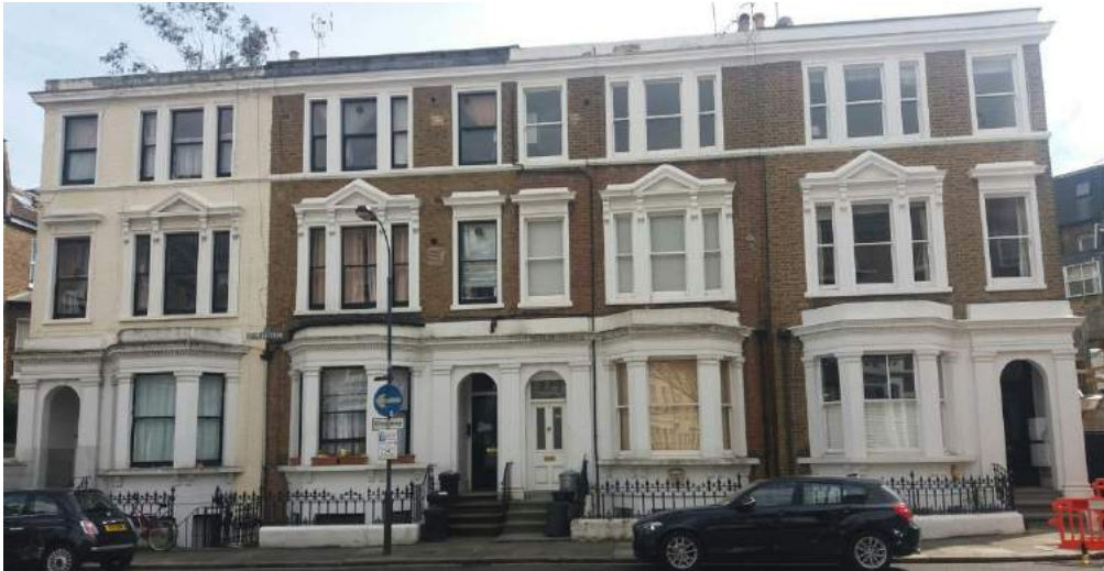
Nos. 1-7 Hazlitt Road. First floor windows with pediments that are typical in this sub area.
