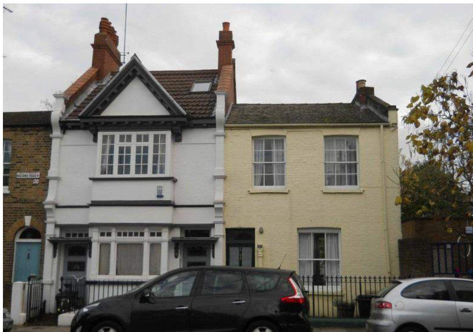
Unusual full height pilasters, no. 42 Masbro Road.
