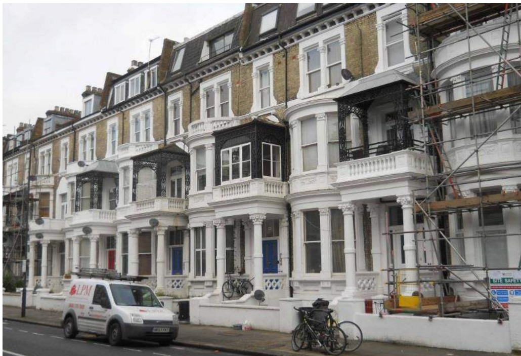
Semi-circular bays and canopies on nos. 116-142 Sinclair Road.
