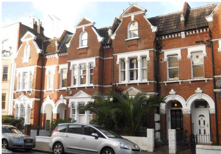
Houses in Addison Gardens, nos. 142-148. Richly detailed facades are further enhanced by planting in front gardens.
