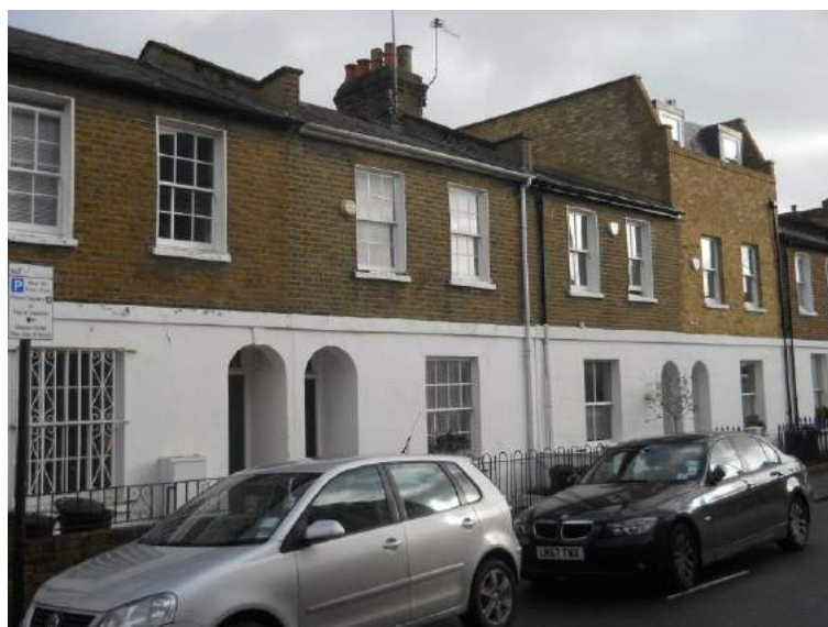
No. 49 Milson Road. Prominent additional floors have disrupted the consistency of the terrace.
