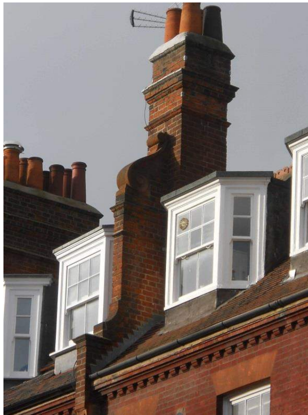
Distinct chimneys on nos. 53-59 and 40-62, Addison Gardens piers with scrolls.
