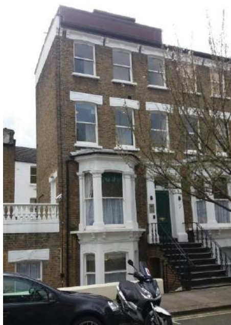
No. 7 Minford Gardens and view through to Westwick Gardens.
