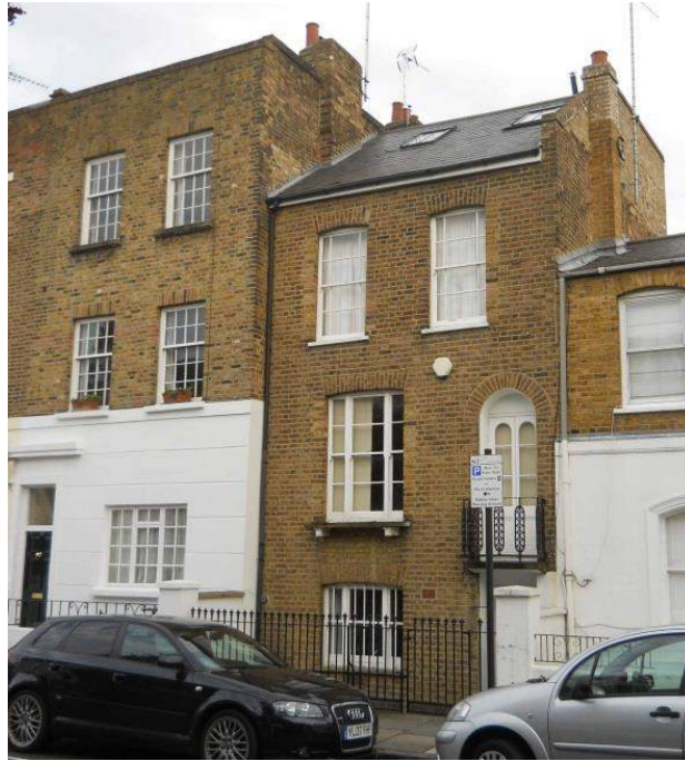
Juliet balcony provides canopy, no. 54 Masbro Road.
